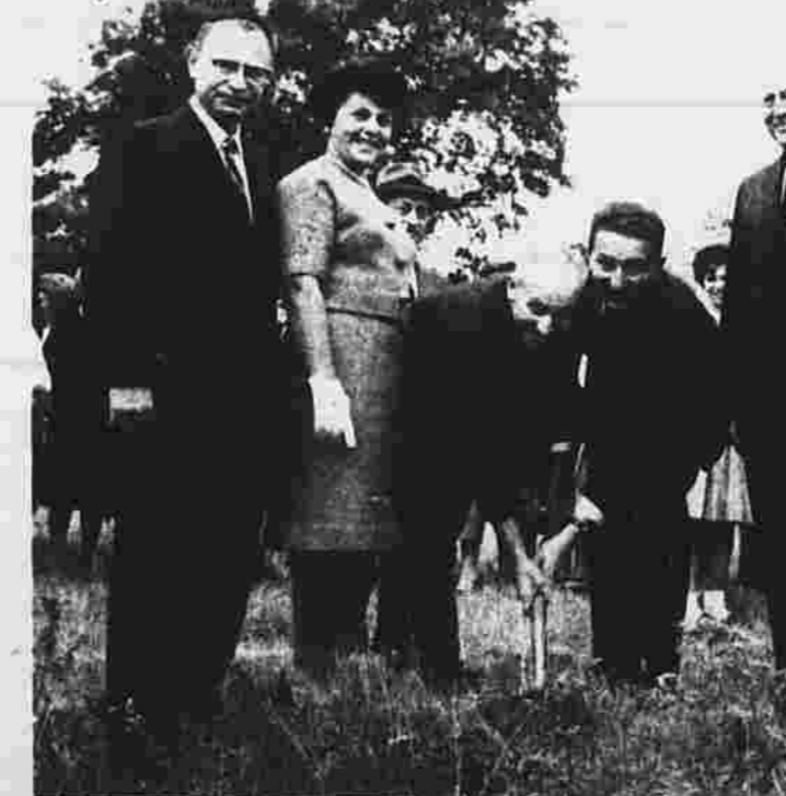
This 1962 photo shows Temple President Phillip Harrison and Philip Bayer, now deceased, holding the shovel to break ground for the temple. Looking on, from left, are Rabbi Wind; Hyalle Hurwitz, then president of the temple sisterhood; Building Committee Chair-
